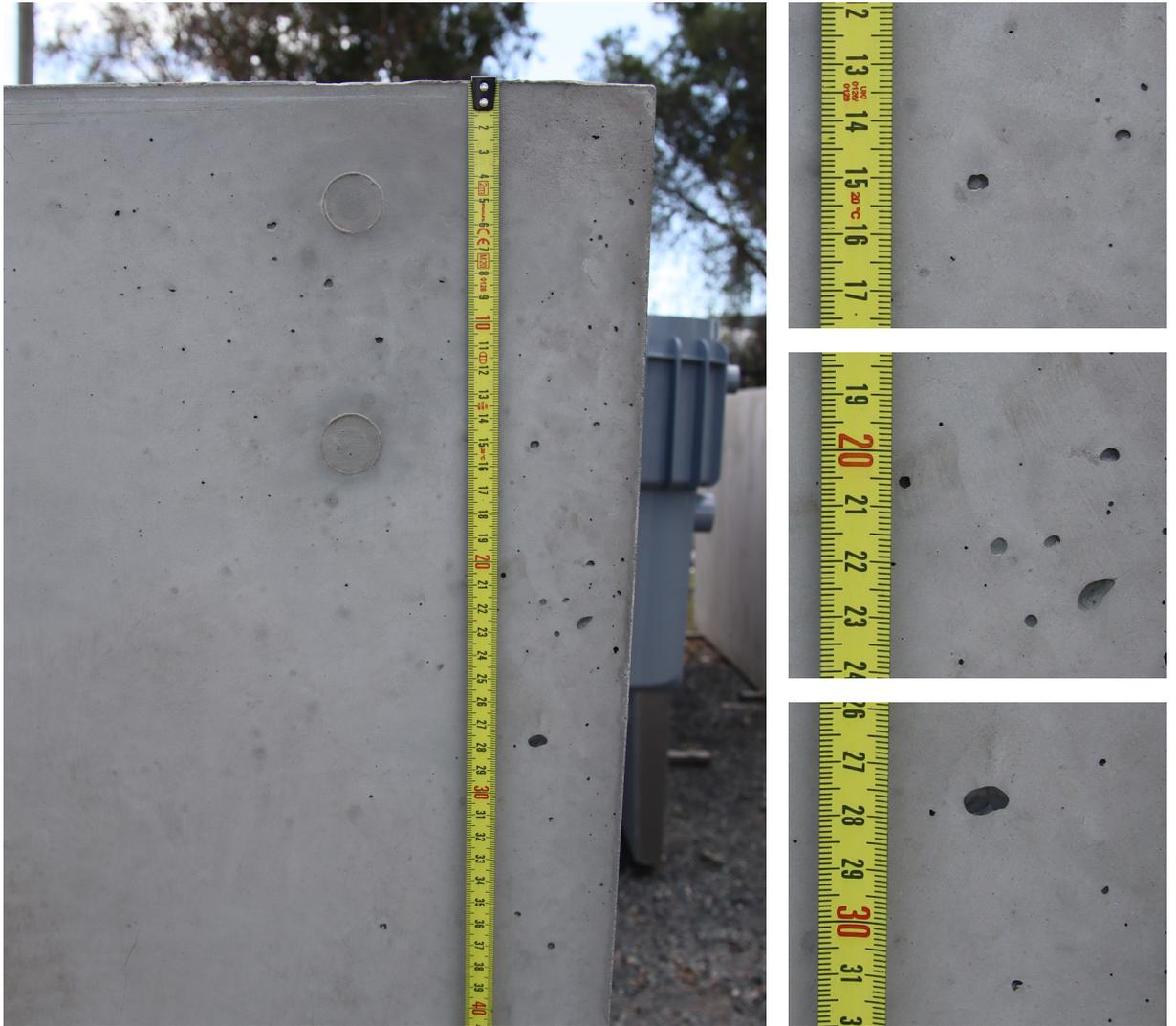
Note: The bubbles that show on the underside surfaces of stairs etc are normal and not visible in most installations. These are unavoidable due to mould design and have no impact on the overall structure of the pool.
