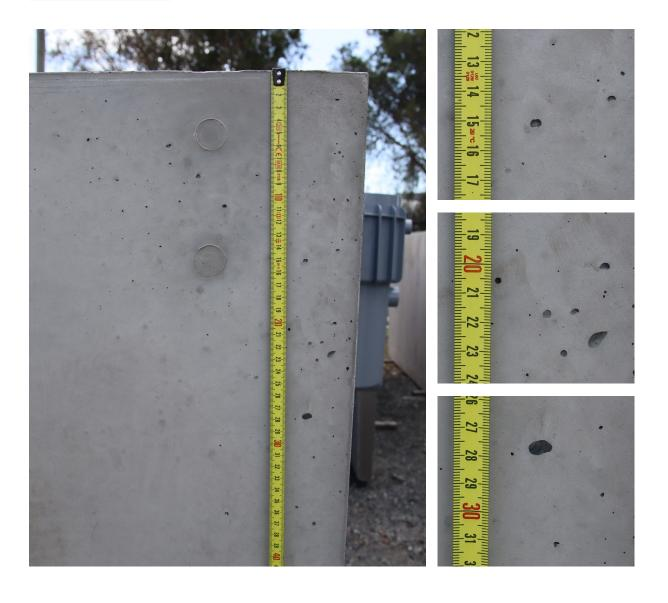
Note: The bubbles that show on the underside surfaces of stairs etc are normal and not visible in most installations. These are unavoidable due to mould design and have no impact on the overall structure of the pool.
